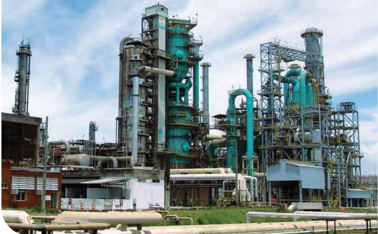
REVAP FCC unit that received the regenerator cyclone and refractory cement
