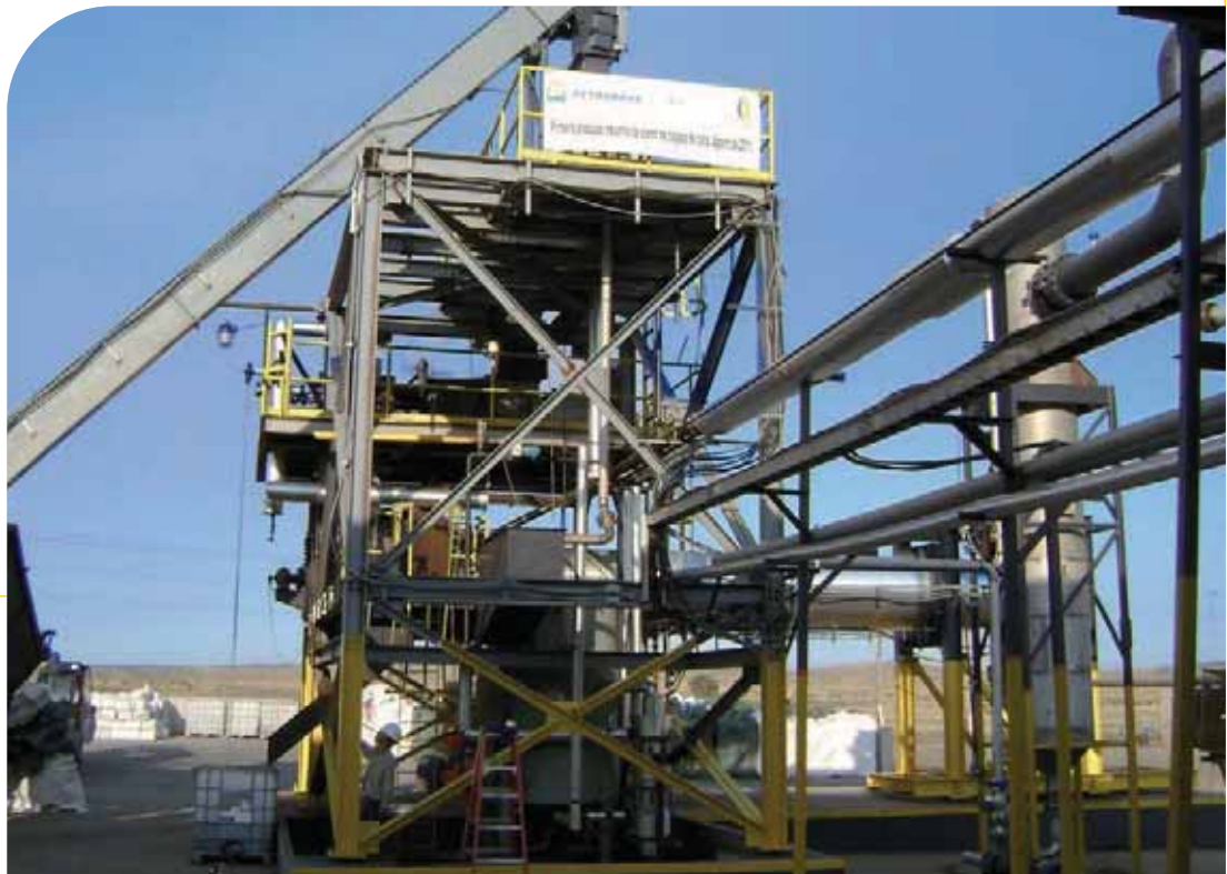
KLE demonstration plant of ethanol production from sugarcane bagasse in Upton, Wyoming (USA)
