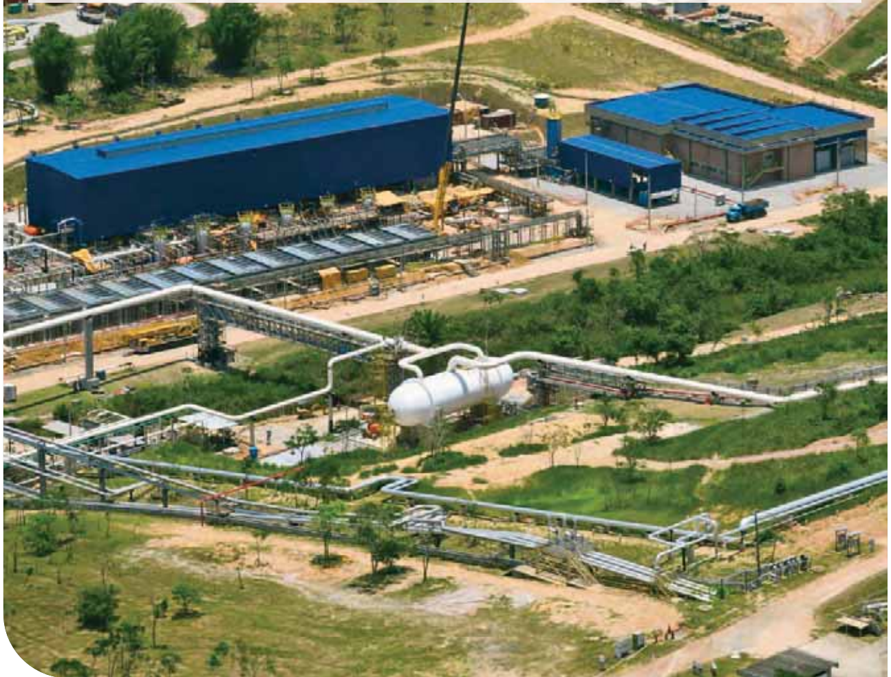
Cabiúnas Terminal, which will have new units to receive gas from the pre-salt region of the Santos Basin
